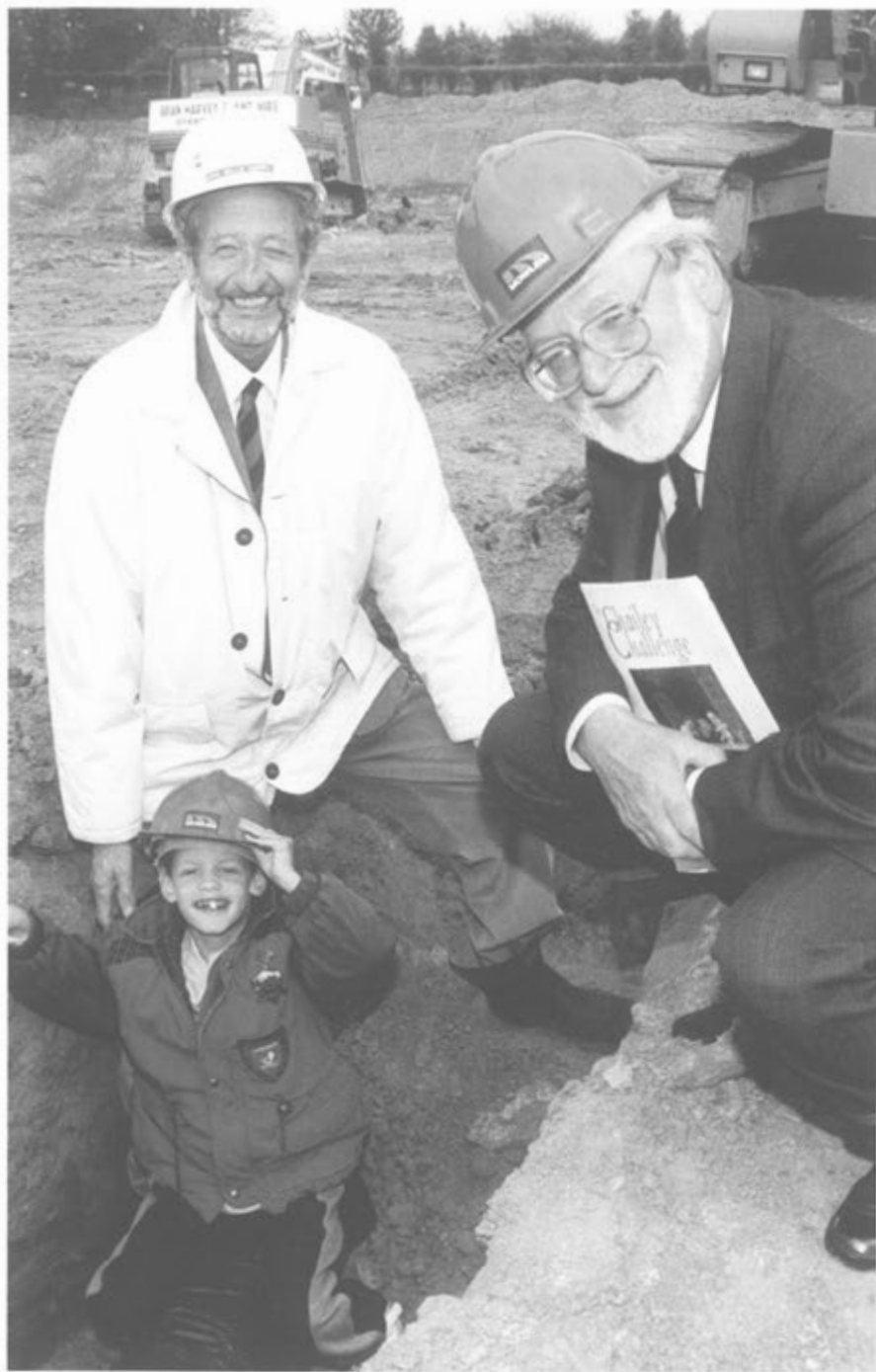
Realising the dream: Friends' chairman Clifford Dann (right) at the Westfield site with John Wells-Thorpe, chairman of the South Downs NHS Trust, and young Timmy Henry, so thrilled to watch the progress of the project that he was declared 'foreman of the works'.
